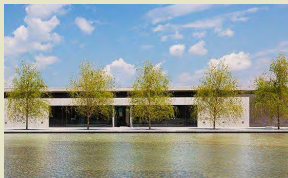
Above: The Clark Art Institute in Williamstown, Massachusetts
